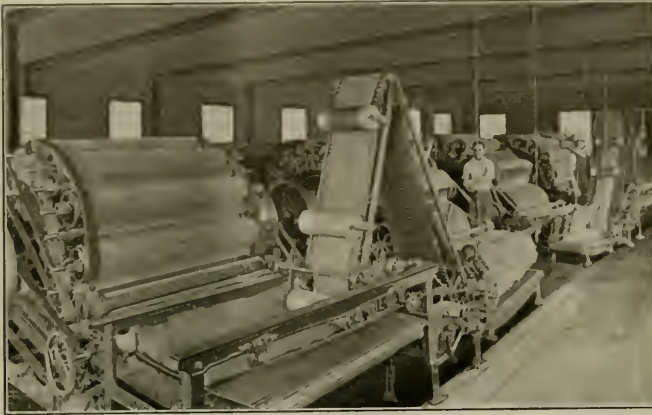
SECTION SHOWING CARDS IN SPINNING DEPARTMENT.
